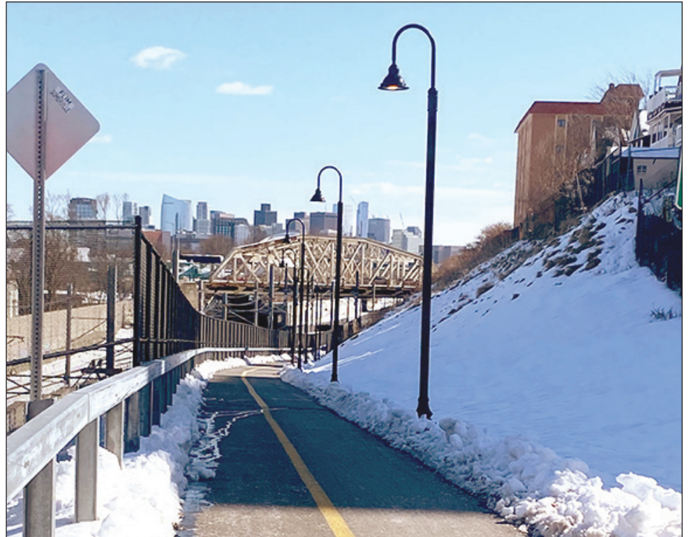
Bids are being accepted for improvements to the lighting on Somerville's Community Path.
